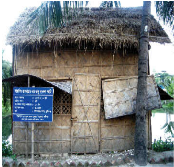
Simple low cost thatch house, a storage facility, saved hundreds of tons of potato of poor farmers
