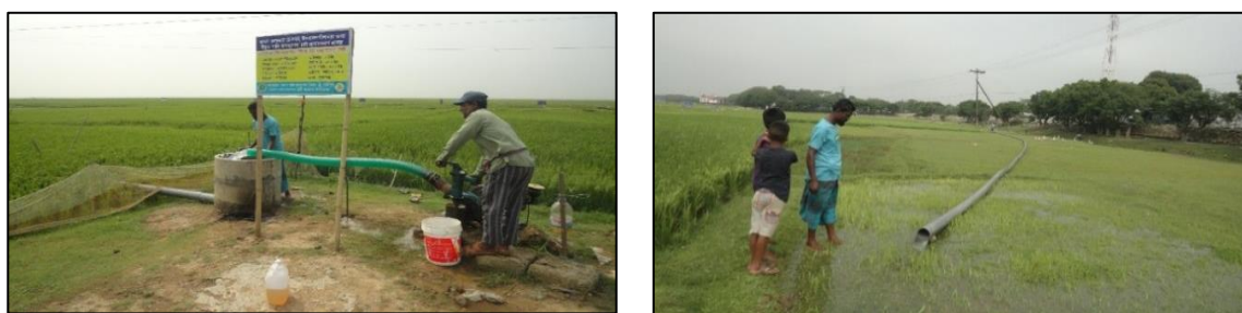
Fig. 2: Surface-laid PVC pipe irrigation water distribution system (a) Stand tank (b) Outlet
