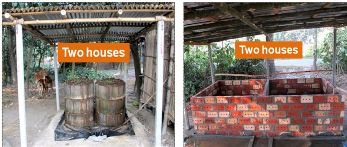
Fig. 4. Cemented ring (1) and brick made (2) house of Tricho-compost production
